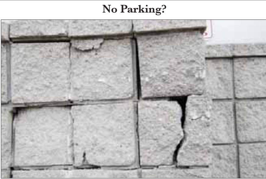
The Jacksons Texaco in Homedale suffered some Thanksgiving day damage shortly before 3 p.m., when a customer's brakes failed and a Ford Bronco struck the west side of the building. The impact dislodged and fractured the stone blocks forming the wall of the store, and possibly damaged the studs within the wall as well, according to a Homedale Police Department report.
